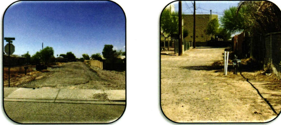
Figure 9: Unpaved Alleys and Streets
