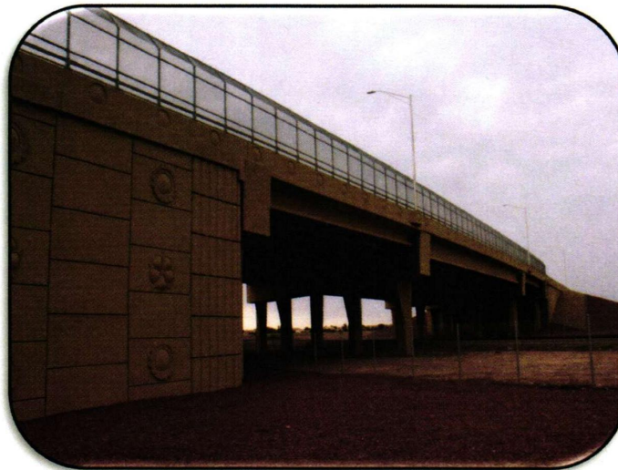
Figure 22: Freeway Overpass Art
